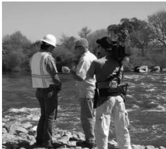
Huell Howser interviews Vernon Silva of Ford Construction Company as the crew builds up levees on the San Joaquin River.
