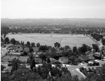
ETWD Regional Emergency Reservoir 275 Million Gallons
